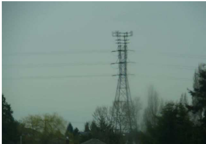
Cell Site on Hydro Tower
